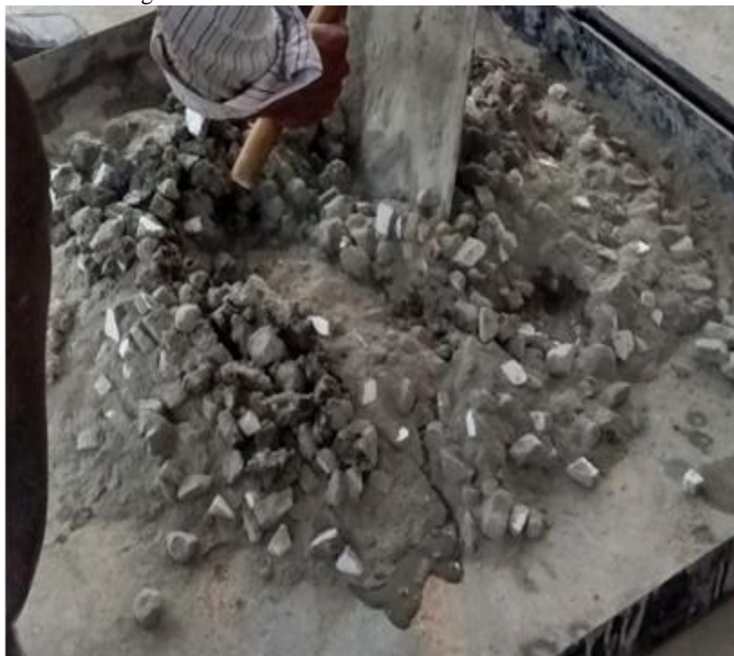
Fig 8: Mixing of concrete
